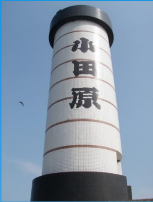
Odawara second breakwater lighthouse (Odawara-city)
