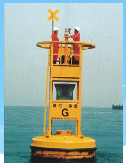
Light buoy inspection
